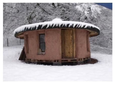
A place apart – the finished poustinia hardly needs any heating thanks to straw bale construction
